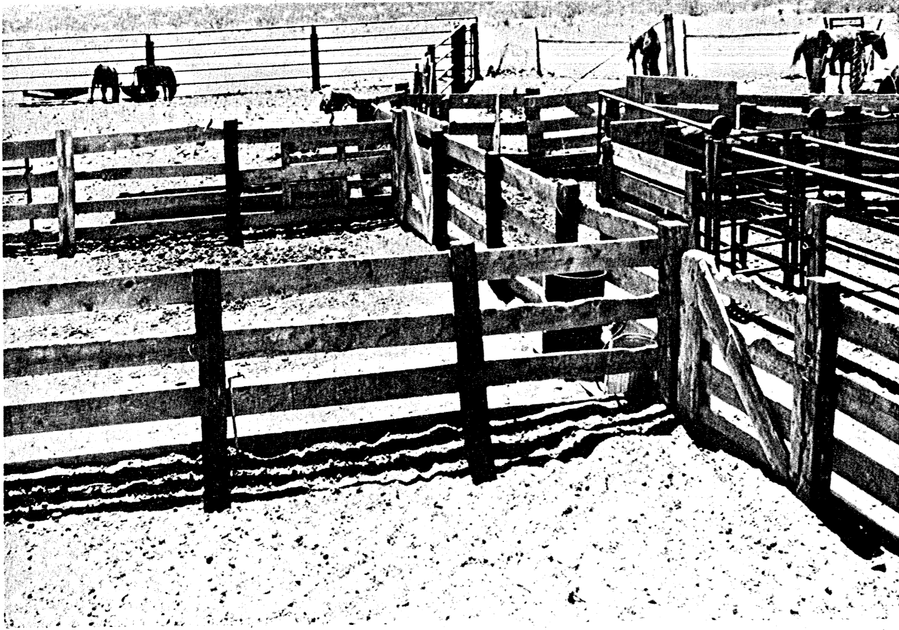
READYING THE ARENA—Repairs and additions have been completed at the present NMSU rodeo arena in preparation for next week's rodeo. Old pens at the arena have been repaired and new ones have been added. New pens at the arena were constructed from pipe to be used in the building of the new arena and will be transported to the new site when construction begins. (PHOTO BY BARRY)
