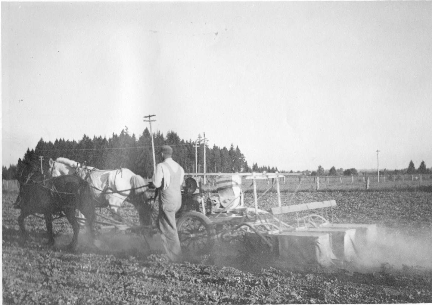
Figure 3. Side View of Duster Used in Experimental Dusting of Strawberries
